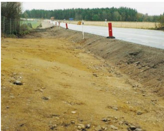
Improving roadside areas increases road safety. Hazardous obstacles such as rock-faces, posts and trees are removed in order to prevent injury in an accident.
