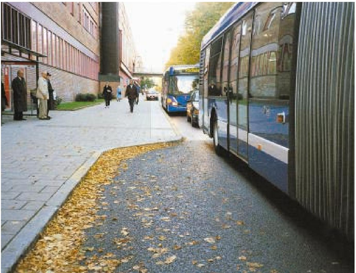
This kind of lay-by bus stop offers several advantages in built-up areas, e.g. increasing road traffic safety, providing space for waiting passengers and increasing car parking space.
